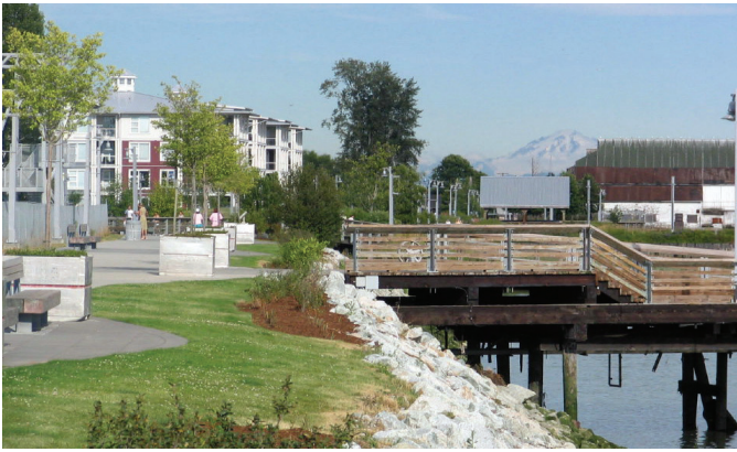
The development of the BC Packers land in Steveston demonstrates how the historical embankments of the Fraser River are changing from industrial uses to high-density residential uses.
